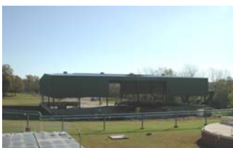
The roof built over Hopewell Regional Water Treatment Facility sludge pad reduced stormwater contamination by nearly eliminating sludge runoff.
