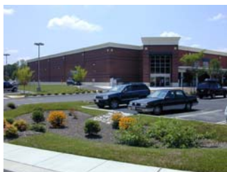
Ukrop's Super Markets bio-retention area traps and filters runoff from the store's parking lot.
